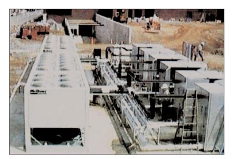
At the left of the photograph are the two air cooled screw machines which provide refrigerant to the six slurry generators located on the right of the photograph. One screw machine drives three 64-ton slurry generators. The storage tank is located below the equipment with the tank cover serving as the platform for the equipment. The slurry drops directly into the tank below as illustrated by the above schematic.
