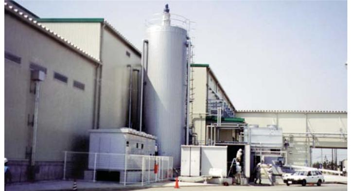
ORE-100 units installed at a dairy processing plant in Japan. The use of a silo ice-storage tank saves expensive land.
